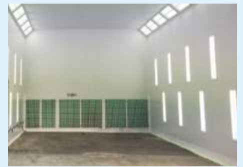
Air exhausted by rear wall
